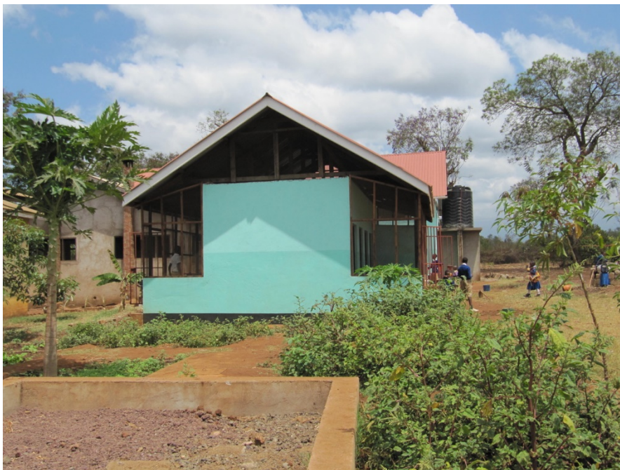
New toilet block
