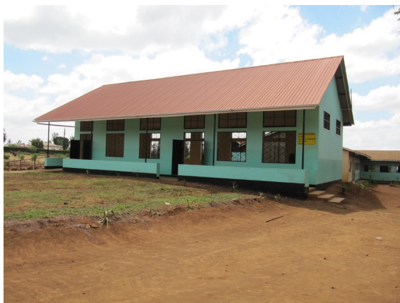
New classroom block
